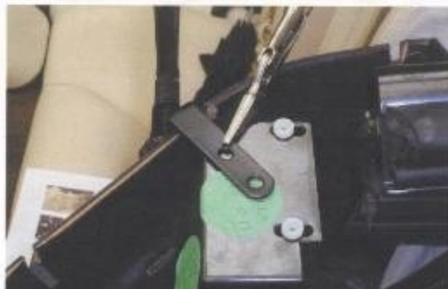
Fig:6 View showing placement of passenger's side larger piece of angle iron prior to drilling.
